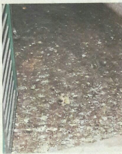
A rooftop room that had attracted pigeons to roost there. The space is filled with droppings and has a bad odour.
